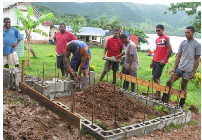
Helping to lay the foundations of the concrete stands
