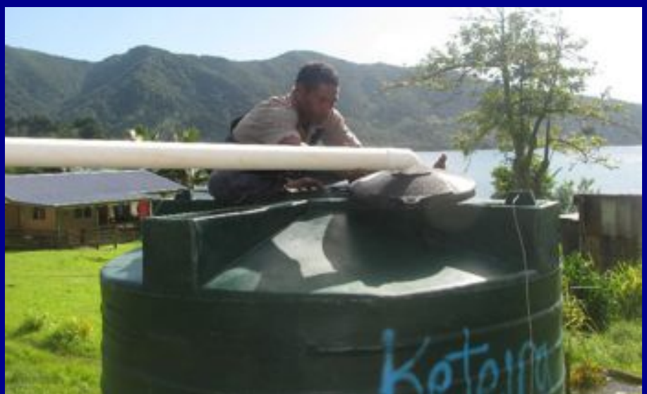
Reinforcing the strainer on the water tank in Keteira village.
