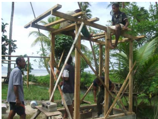
The team building one of the shower houses
